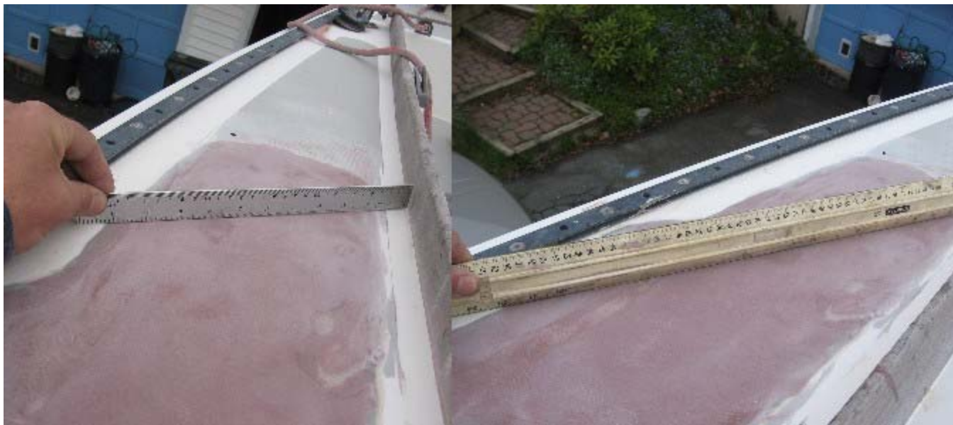
Checking for high spots
