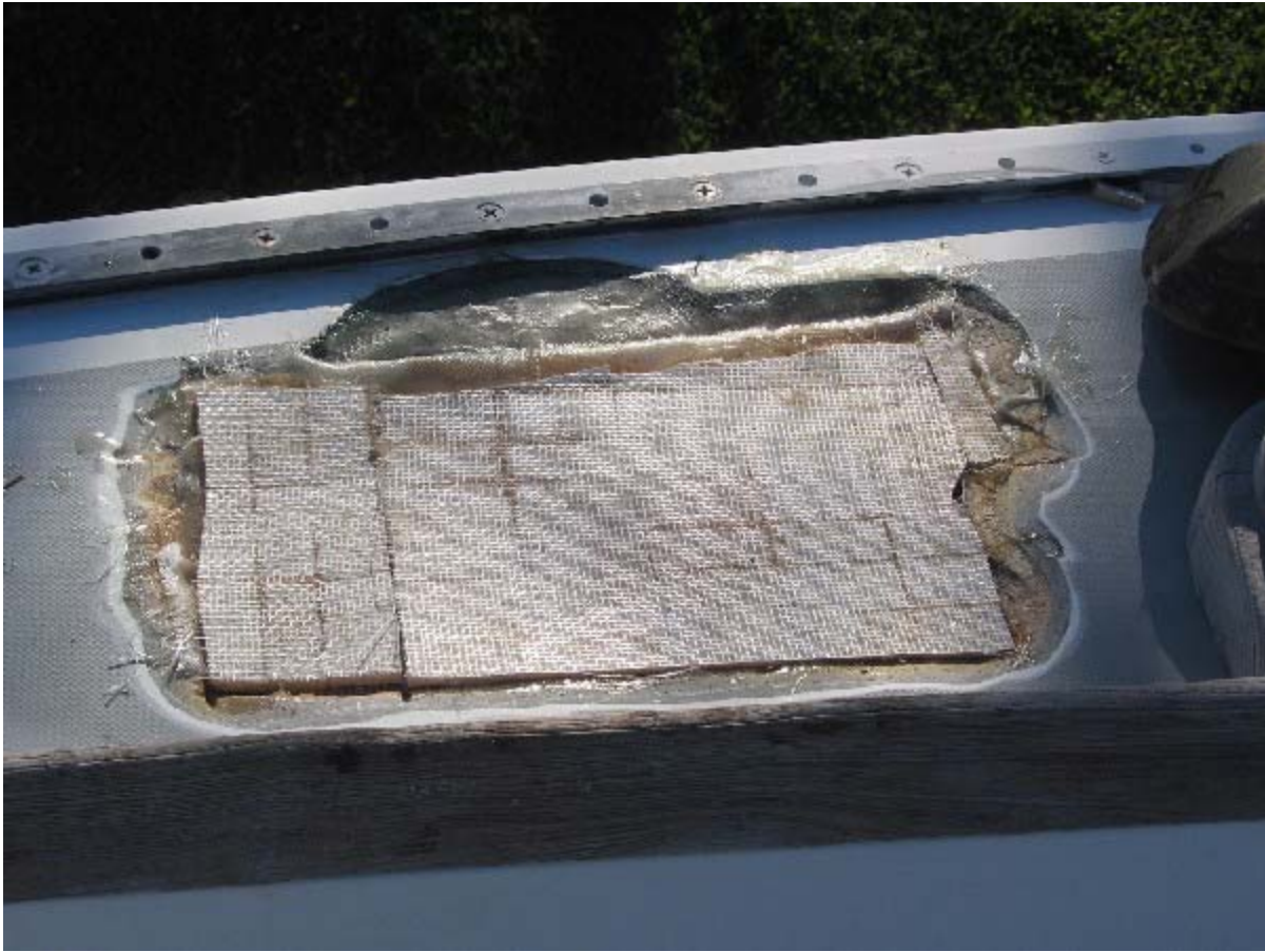
Core Material Epoxied in place in the second area.
