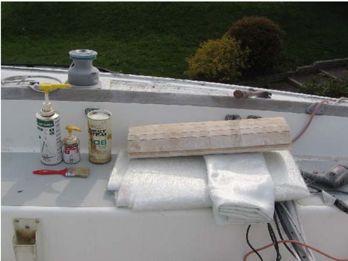
Materials to use. East System Epoxy resin and hardener, West 406 adhesive filler, glass cloth, end grain balsa
