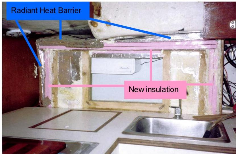
I used expanding foam to fill in every void and gap in the insulation that I could find or even imagine might exist. To get foam to the rear of the box, I stuck the spray tube of the foam can inside one end of a long piece of flexible plastic tubing and taped the other end of the tube to a stick
